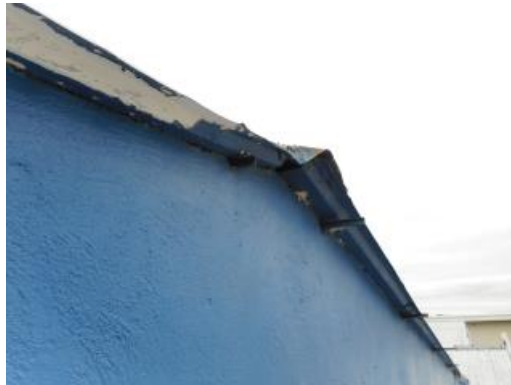
Roof Tie-in to CMU Wall Damage
