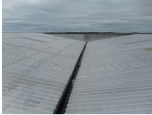
Corrugated Metal Roofing and Box Drain
