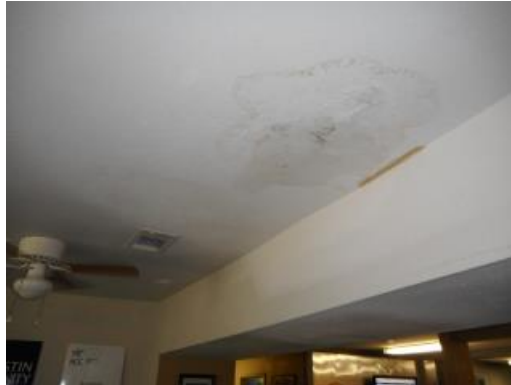
Interior Water Infiltration
