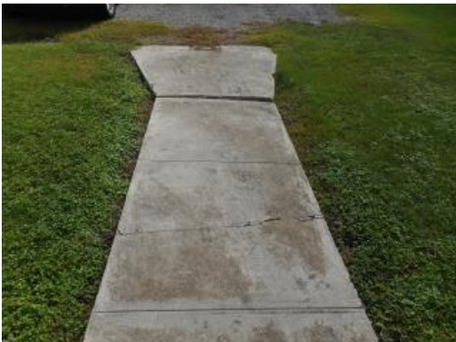
Sidewalk Cracks
