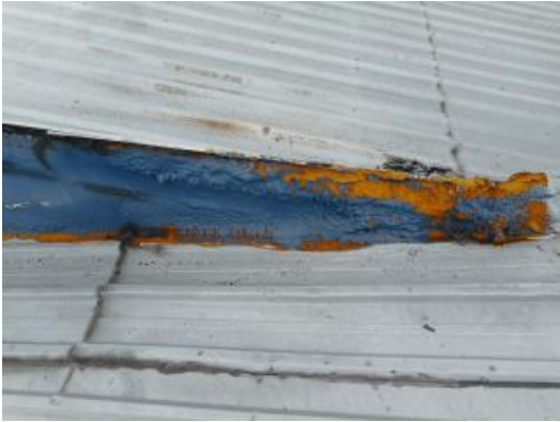
Roof Flashing Failure (South wall above entrance)
