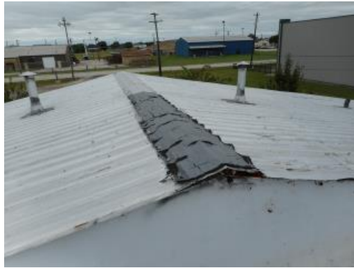
Roof Ridge Damage and Patch
