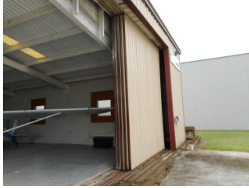
Exterior Sliding Hangar Doors
