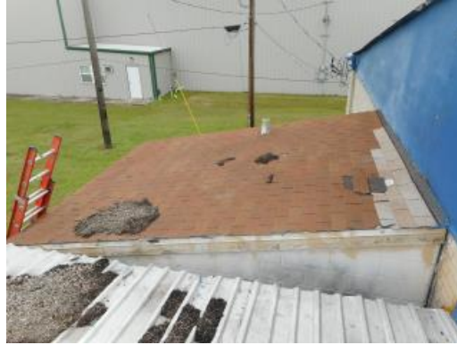
Restroom Roof (Note: No flashing)
