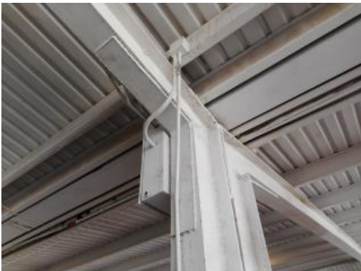
Structural Column Reinforcements
