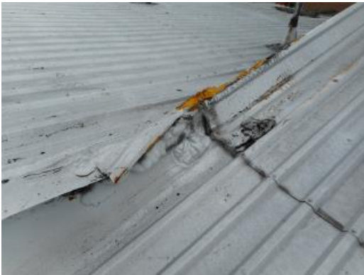
Roof and Flashing Damage (South side)
