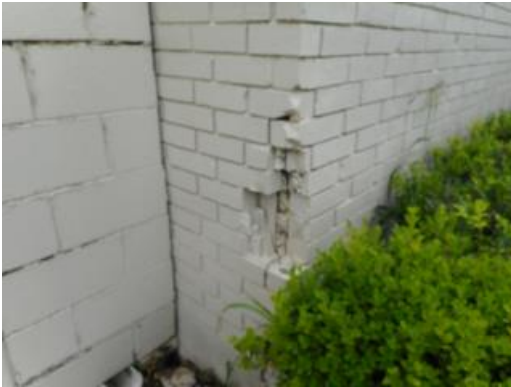
Exterior Brick Veneer Damage
